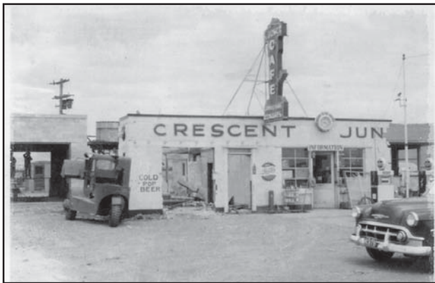
Original building in foreground circa 1956
